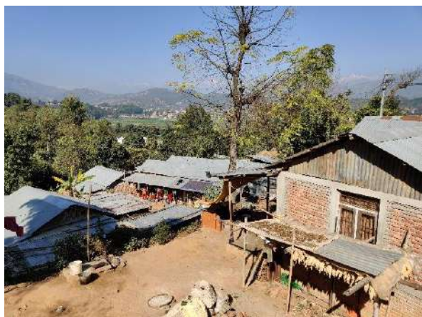
Figure 9 Village under reconstruction (Primary Study)
