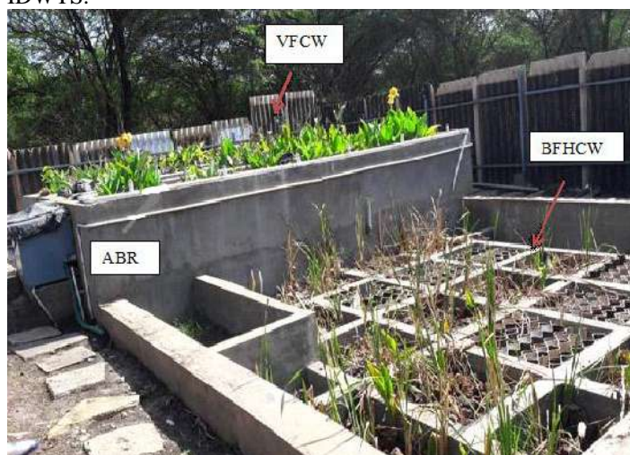
Figure 1: Photographic view of IDWTS at WCE, Sangli.
