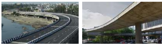
Fig.1. Existing condition of spaces left underneath Flyover (Source: Google)
