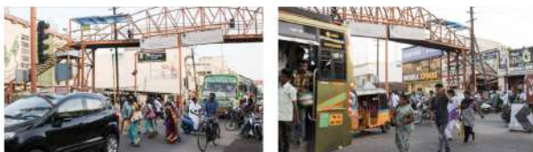
Fig. 7. Foot over bridge in Erode. [23]
