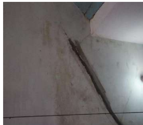
Patchwork with cement plaster
