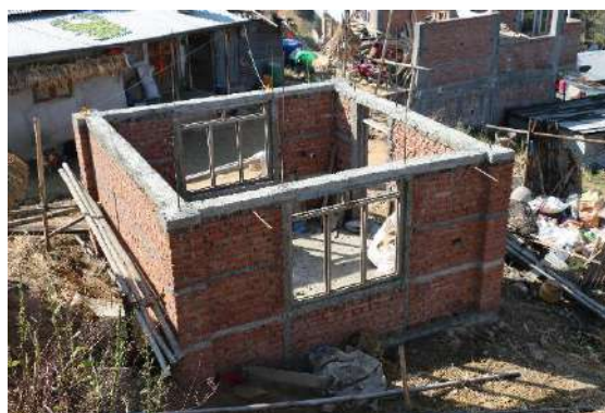
Figure 8 A private house under reconstruction (Primary Study)
