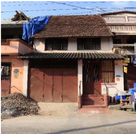
Addition of car porch by taking up the front rooms
