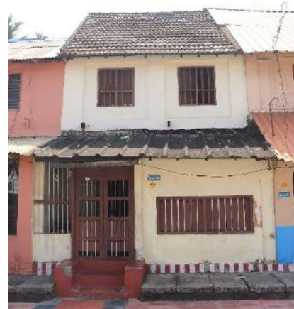
Mangalore tiles replaced by asbestos sheet
